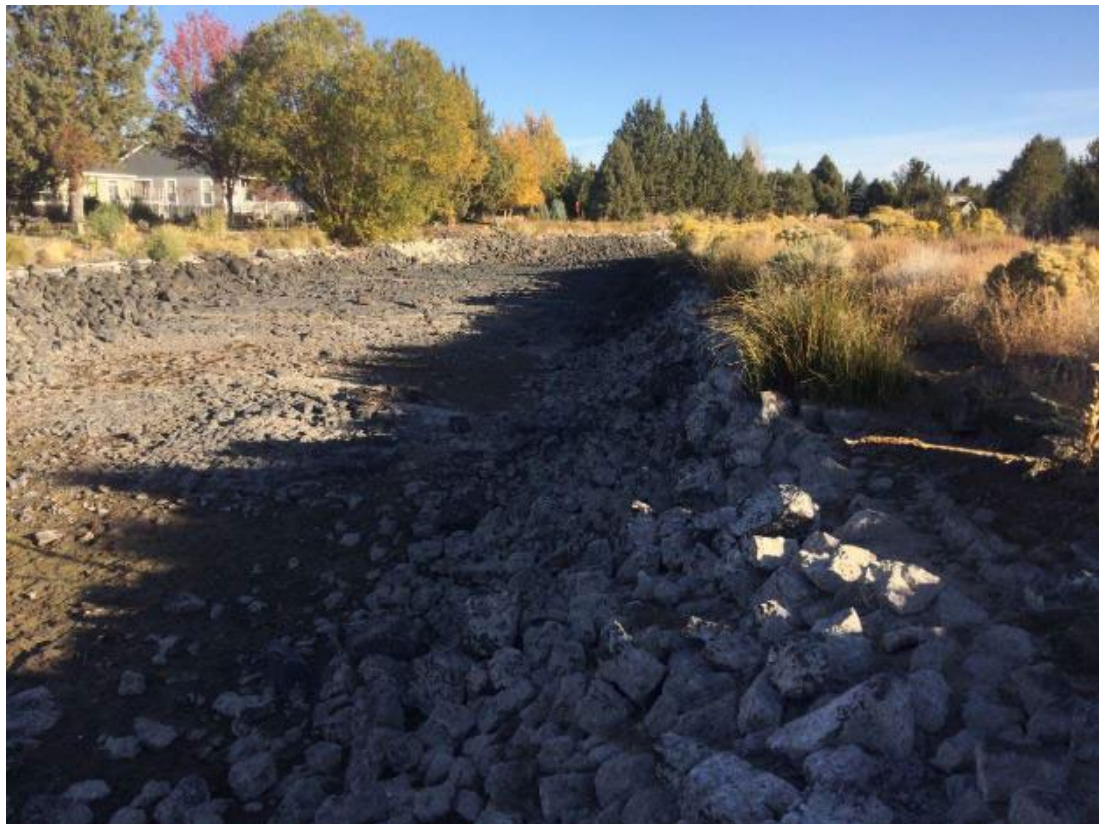
Photograph 1. PBC Alignment in Bend
