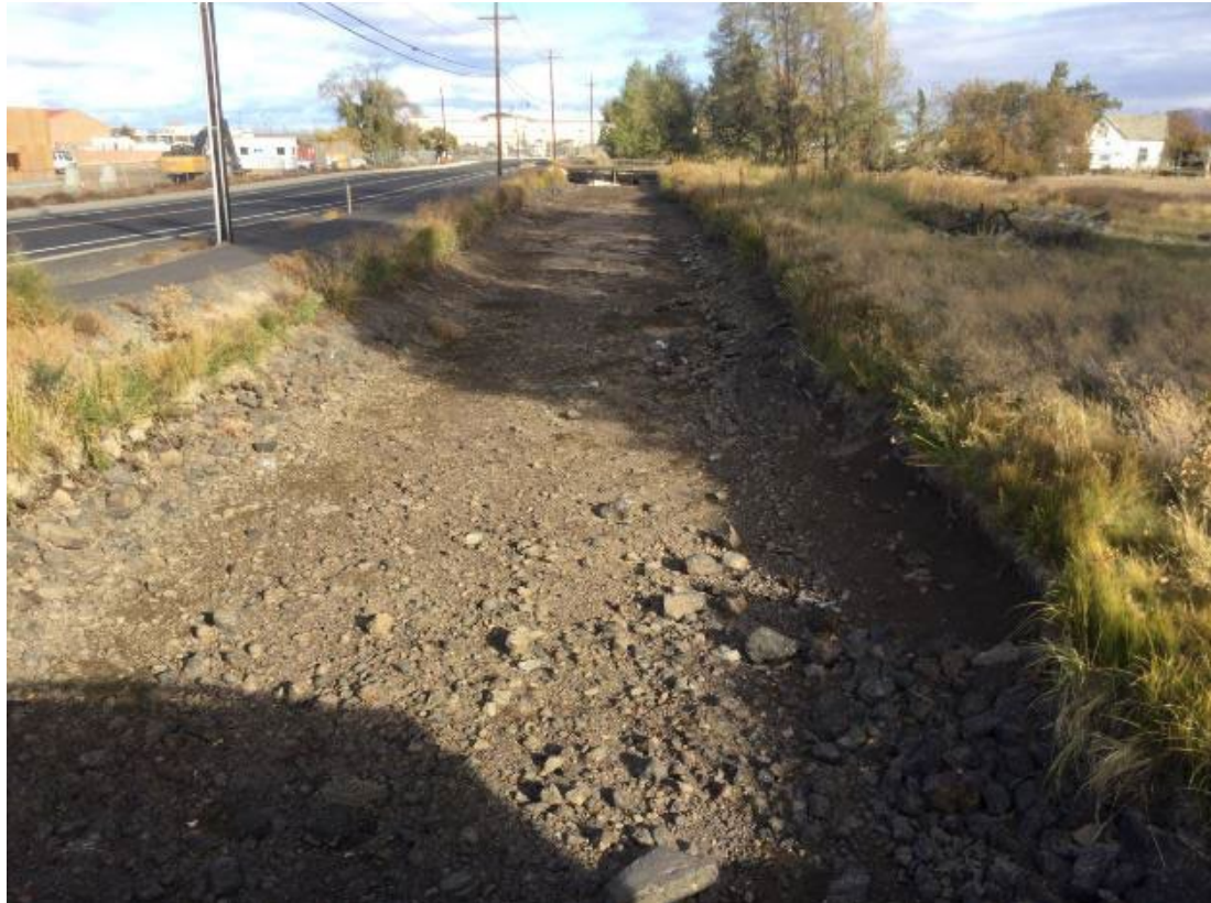
Photograph 3. PBC Alignment in Redmond
