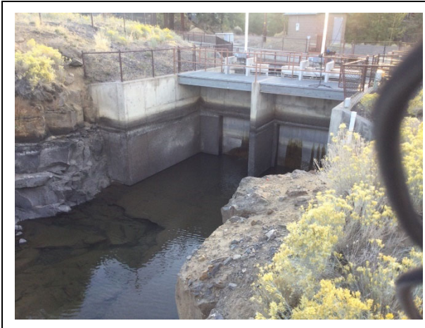
Photo No. 1. View of ODFW-compliant fish screens in Bend.
