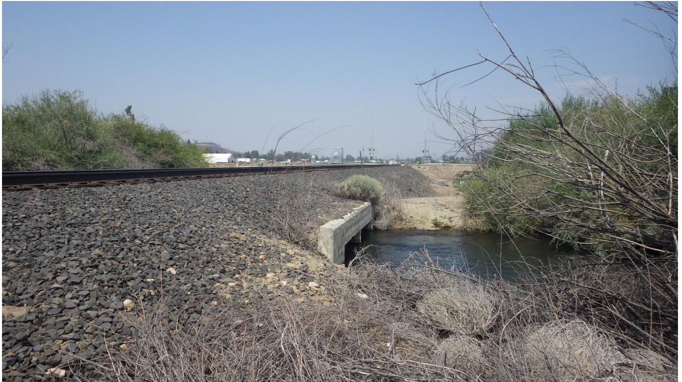
View: OTR/PBC Crossing, Looking NW (G. Kramer, August 2024)
