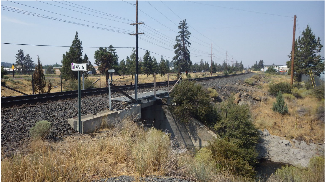
View: OTR/PBC Crossing, Looking Northwest from COID/PBC Maintenance Road (G. Kramer, August 2024)
