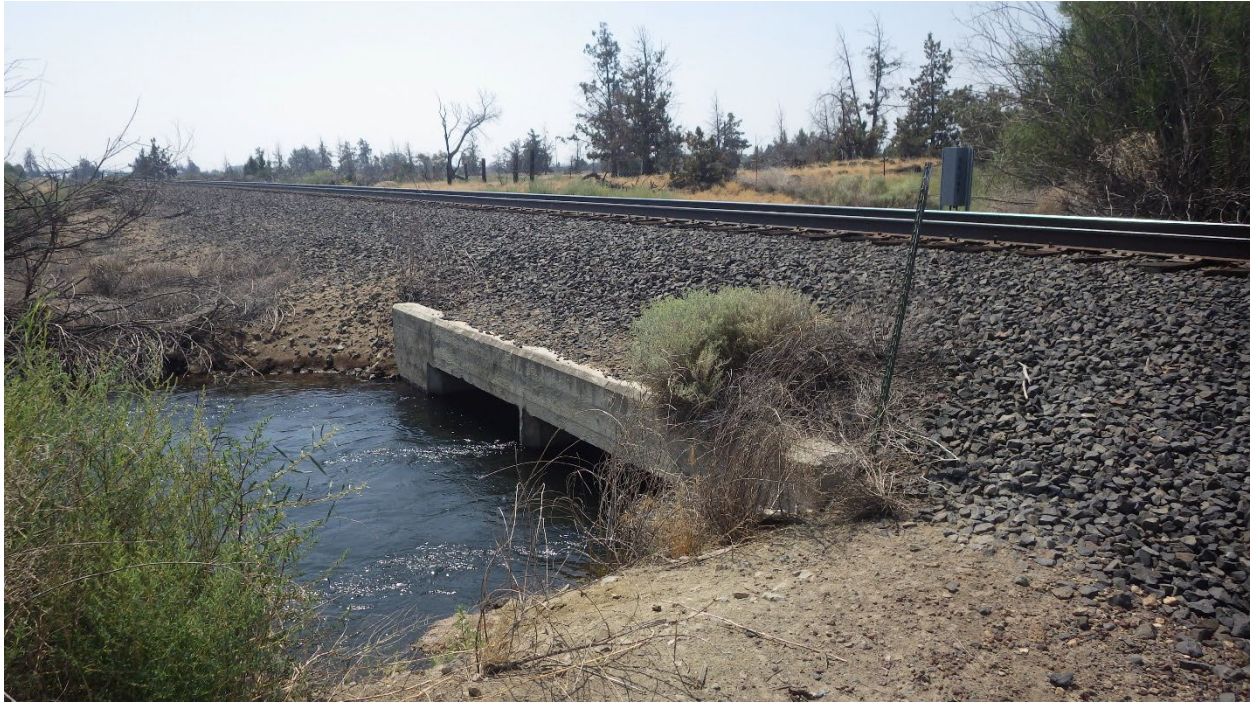
OTR Line, Crossing Pilot Butte Canal near NE King Way, Looking SW (August 2024)
