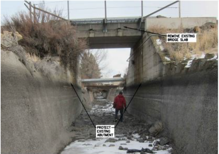
BNSF RAILROAD EXISTING CONDITION
