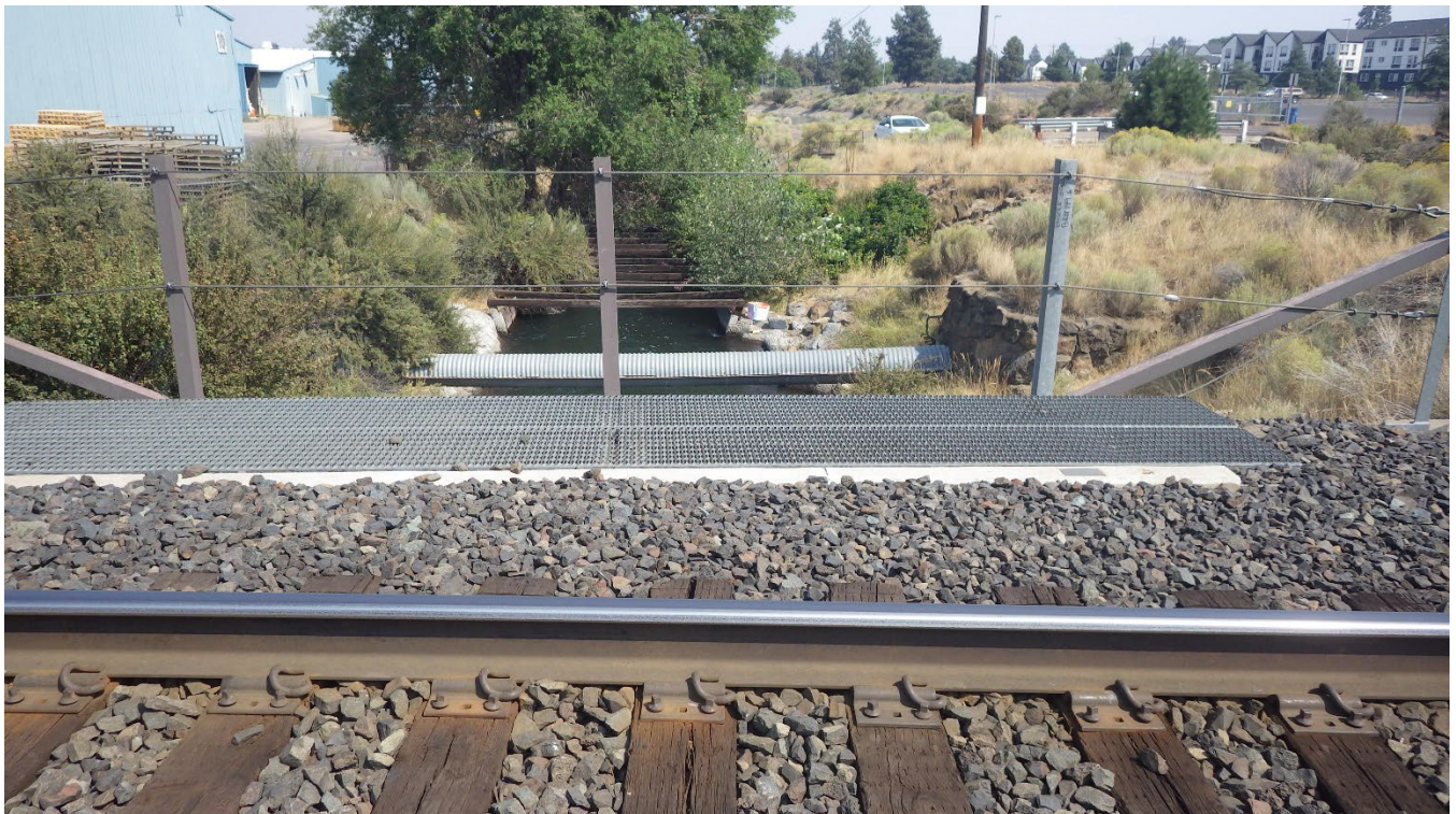
View: OTR/PBC Crossing, Looking East, from OTR Track (G. Kramer, August 2024)
