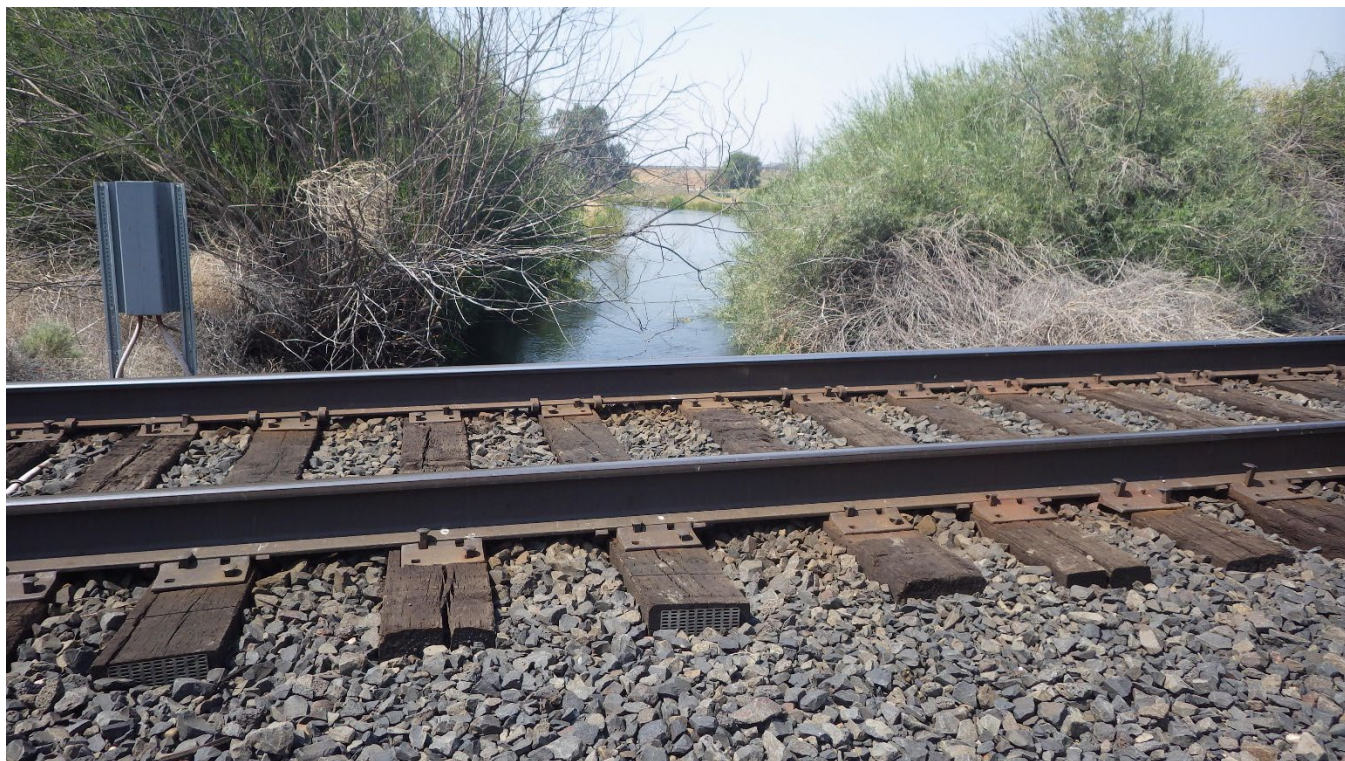
View: OTR/PBC Crossing, Looking West from OTR Line (G. Kramer, August 2024)
