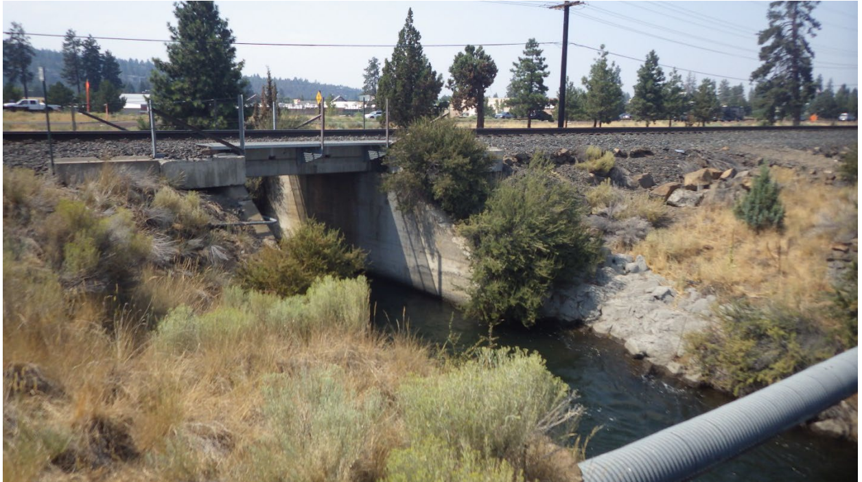
OTR Line, Crossing Pilot Butte Canal near NE Butler Market Road, Looking NW (August 2024)
