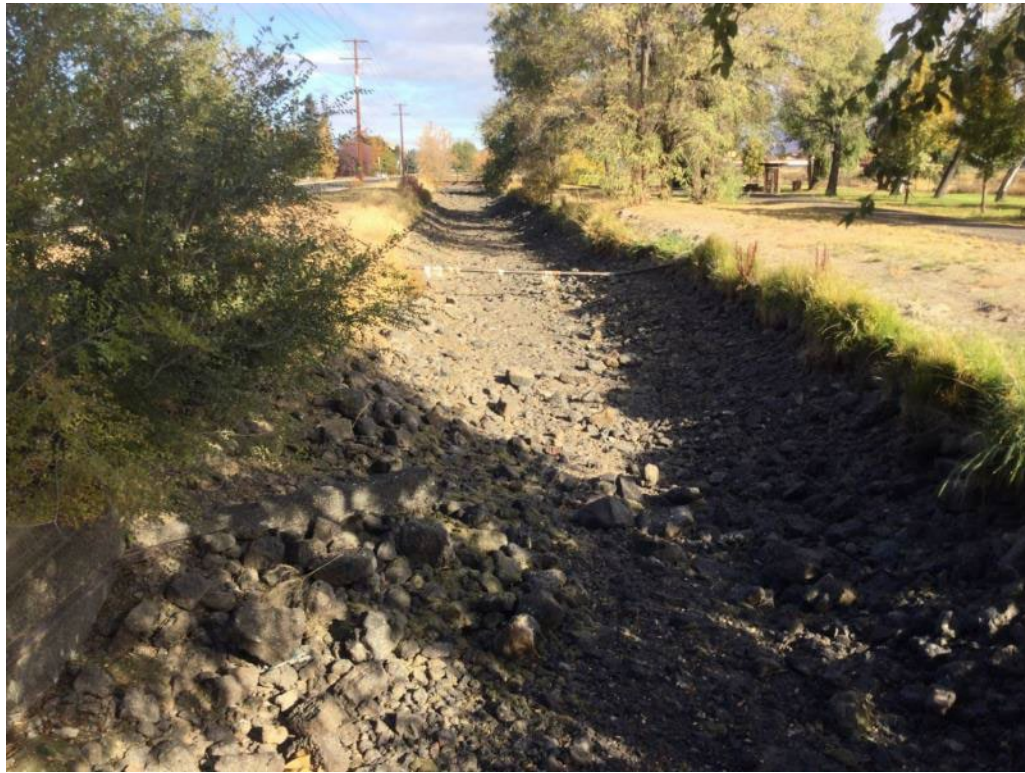
FIGURE 15 Pilot Butte Canal – Downtown Redmond Segment Near NW Fir Avenue (Parametrix, 2021)
