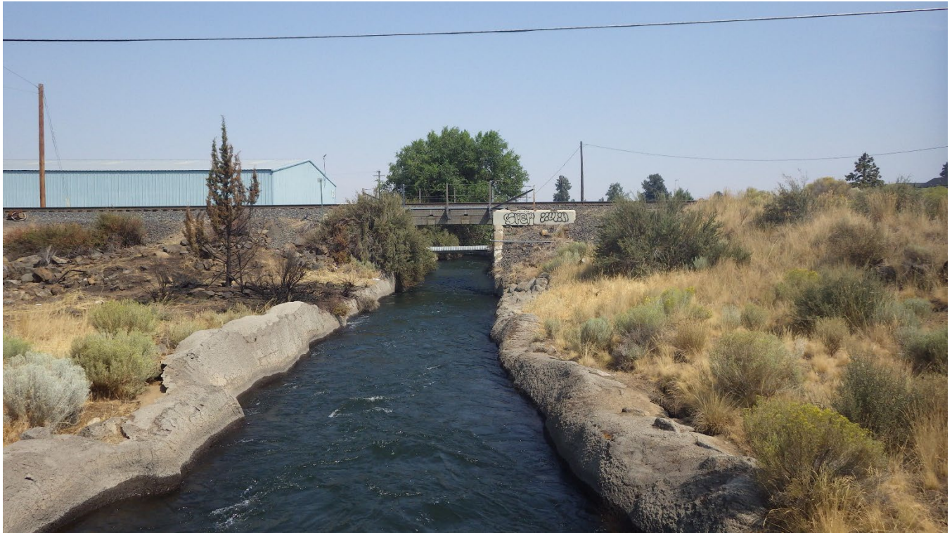
View: OTR/PBC Crossing, Looking East from US 97 Onramp (G. Kramer, August 2024)
