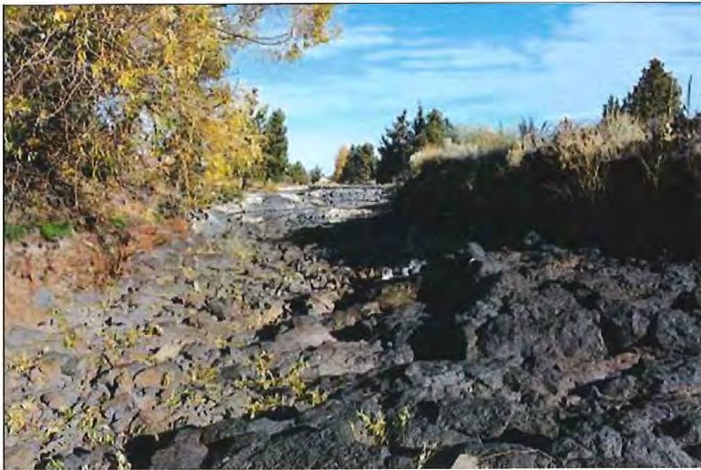
Photo 2 of 19: Segment 1. Irregular, rocky canal bed, looking north.
