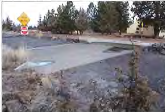
SEGMENT 5: 55' wide by 46' long concrete flow-measuring weir constructed in the canal bed in 2012. Photographer looking northeast.
