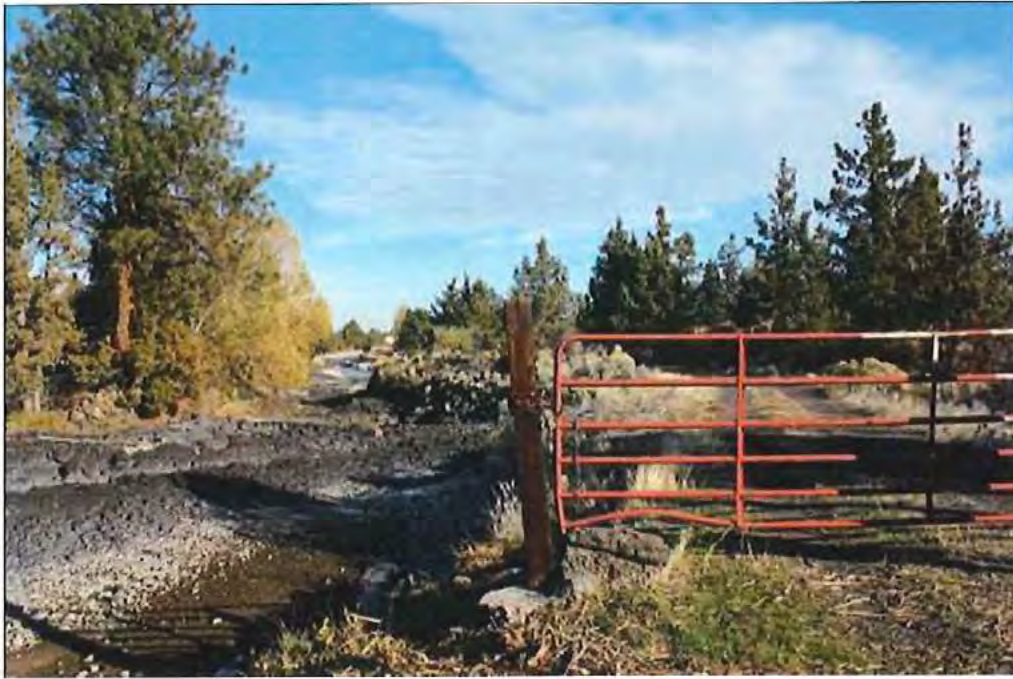
Photo 1 of 19: Segment 1. Highly irregular canal sides and bed; canal curves around solid rock. Metal agricultural gate crosses top of berm at the southern boundary Section 15 and the historic district, looking north.
