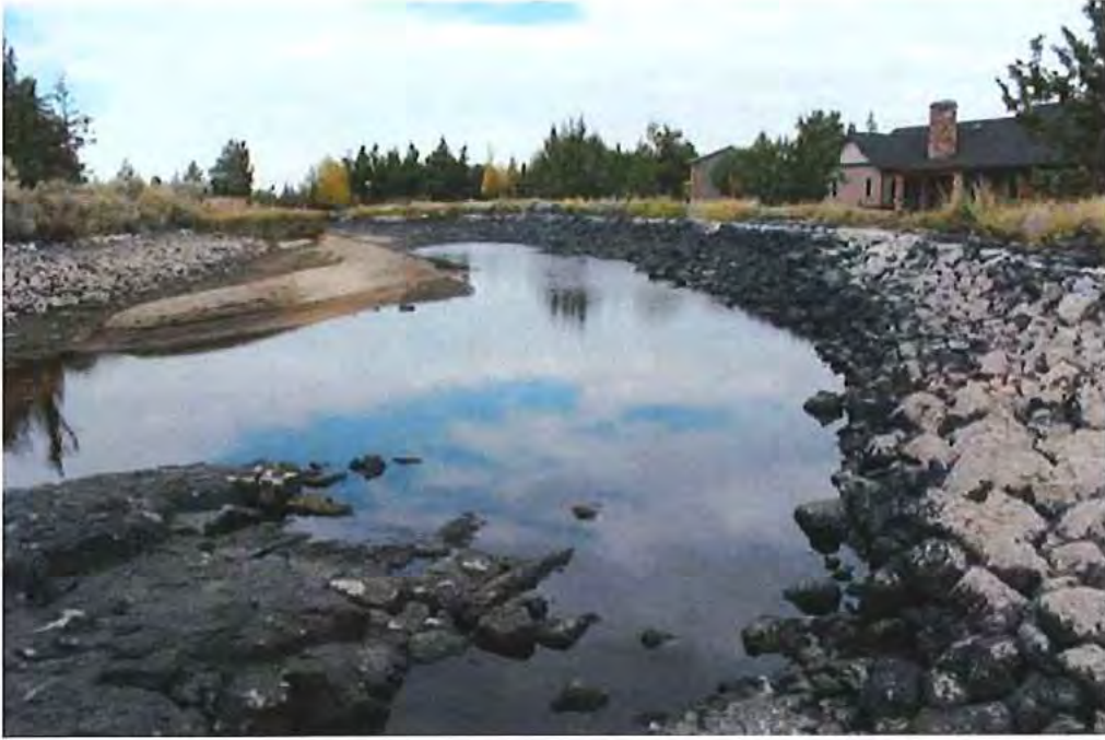
Photo 15 of 19: Segment 5. Canal bed, standing water, lava flow above water level, silt deposits on western bank, looking north.
