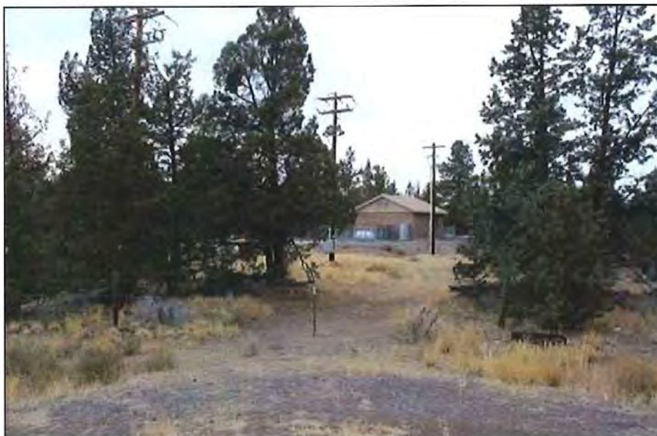
Pipe enters Swalley Hydroelectric Plant, looking west from U.S. Highway 97.
