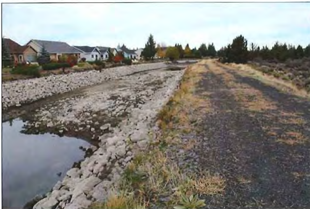
Photo 4 of 19: Segment 1. Relatively symmetrical and straight canal bed. Silt covers rocky bottom. 20-foot wide embankment on east side and consistent side slope on west side of canal, looking north.
