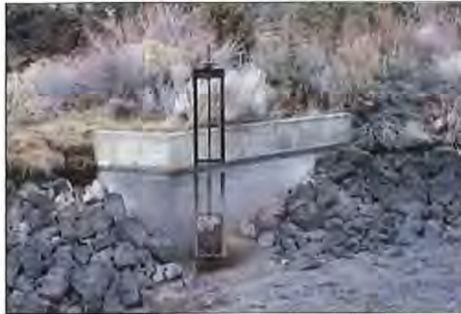
SEGMENT 2: Non-historic metal wheel control, threaded screw lift rod assembly, metal slide gate, concrete headwall and corrugated steel pipe. Photographer looking southwest.
