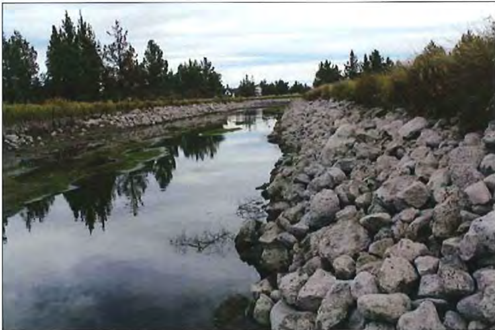
Photo 10 of 19: Segment 3. Canal bed holds water year around at this location; heavily riprapped canal bed and south side slopes; white deposits on rocks; looking east.
