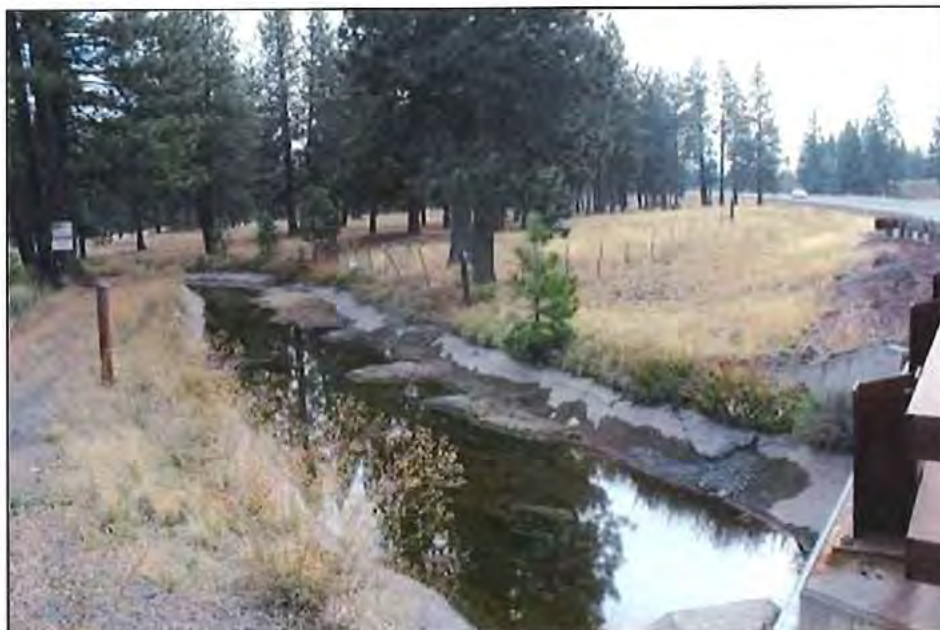
Arnold Canal, lined with concrete, looking east from US Highway 97 near Baker Road overcrossing. Photo taken on October 23, 2015.
