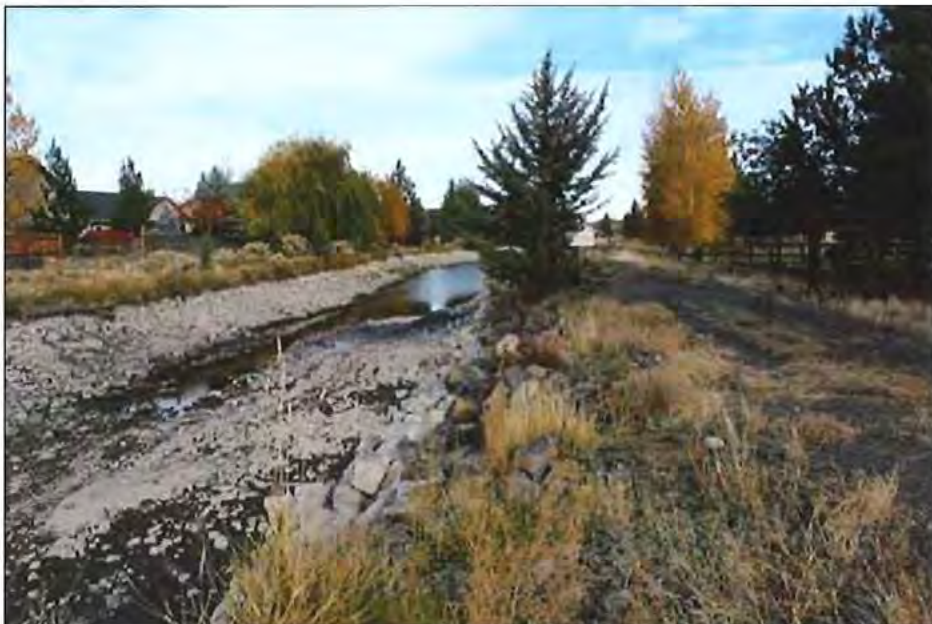
Segment 1: City of Bend on left of canal centerline. At-grade cut on left (west) side of canal; embankment on right (east). Rural county livestock farms on right. Photographer looking north.
