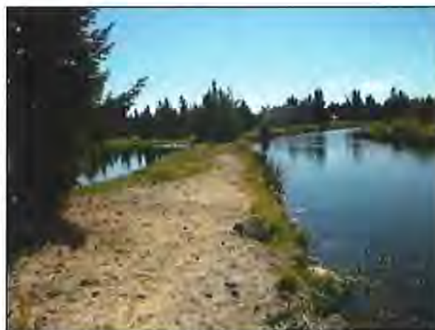
A smooth, deep area in the Pilot Butte Canal Historic District (Cooley Road – Yeoman Road Segment). The irrigation pond on the left is the altered historic Houston Pond. The embankment is about two feet tall in this area. There is no ditch rider road on the embankment. Photographer looking south. 31
