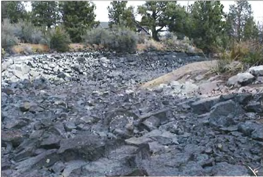
Photo 13 of 19: Segment 4. Irregular, rocky canal bed turning abruptly to east, silt deposit on side of canal bed, looking north.
