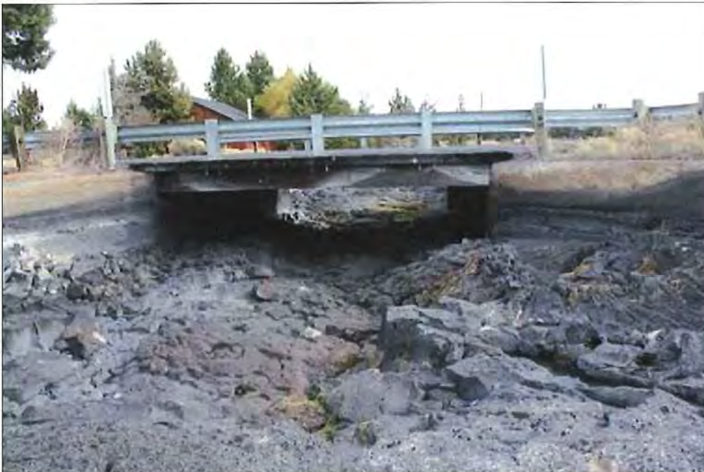
Photo 8 of 19: Segment 2. Canal bed is nearly solid lava flows and narrows to pass under the 1904 Old Deschutes Road Bridge, looking east.
