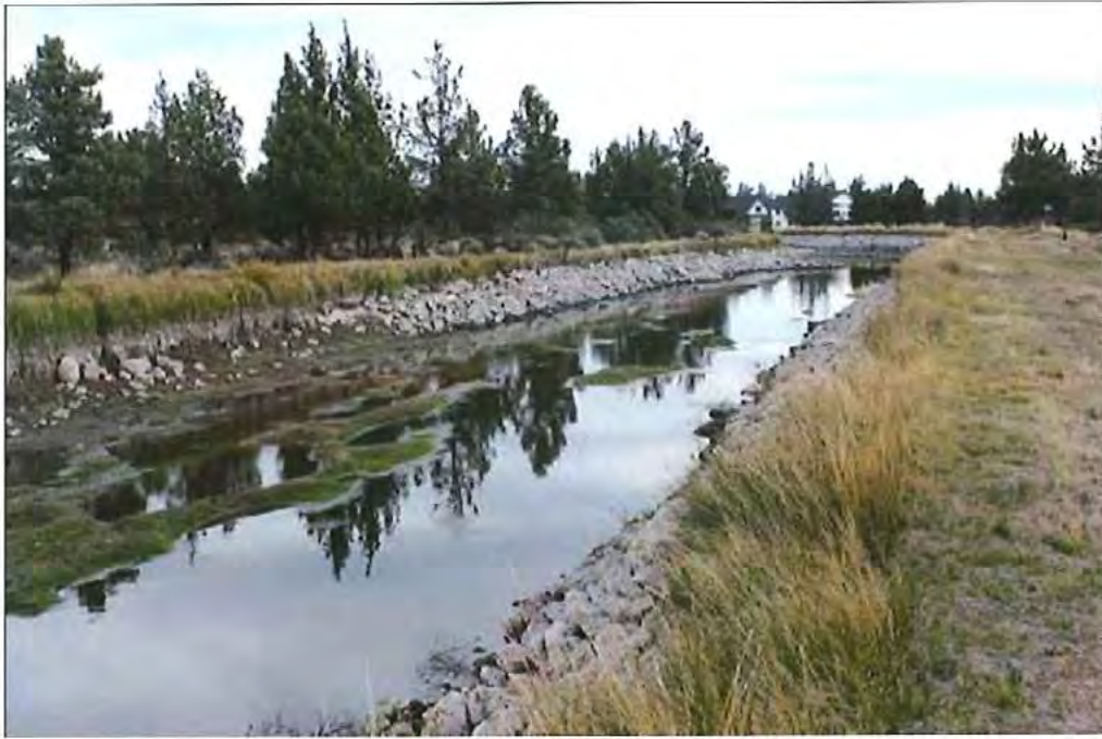
Photo 9 of 19: Segment 3. Canal bed is straight, nearly symmetrical and heavily riprapped. Water stands year-around in this location, looking east.
