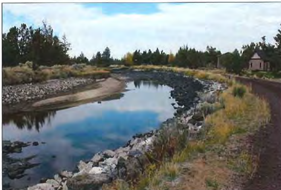
Segment 5: Red cinder covers part of the top of the embankment. This is a gently curving stretch of canal with smaller-diameter loose rock and lava flows in the canal bed. It has riprap on side slopes and standing water with silt piles. Photographer looking northeast.
