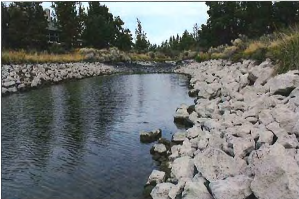
Photo 14 of 19: Segment 4. Canal bed, standing water, heavy riprap, looking north.
