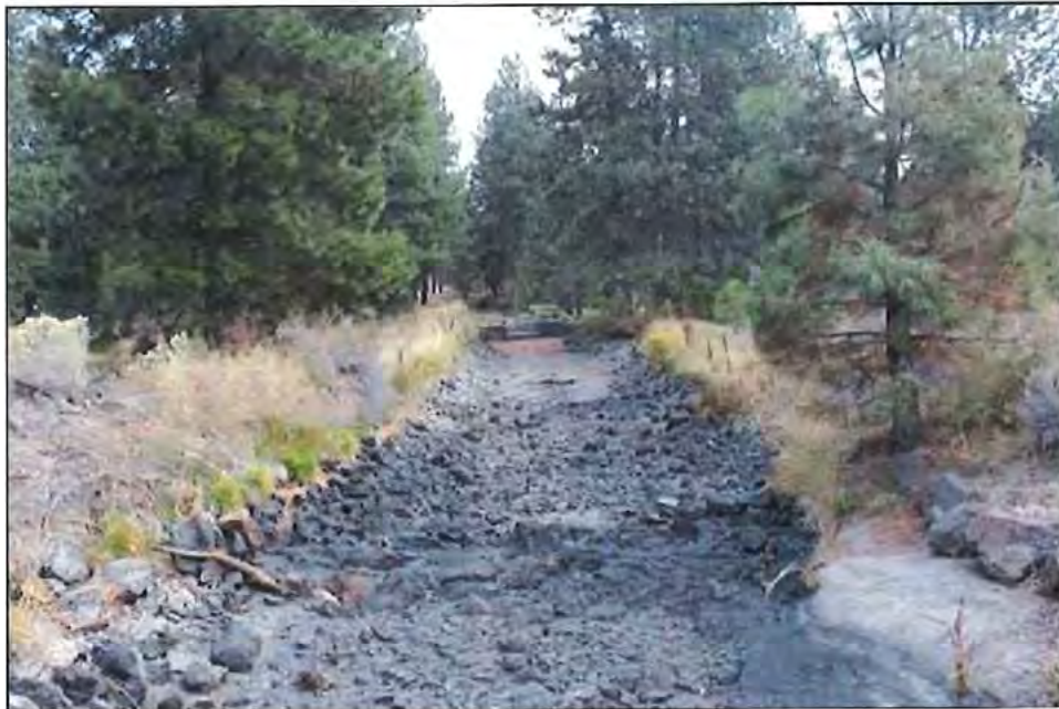
Arnold Canal looking west to east in direction of flow from Brookwood Boulevard near the source, the Deschutes River. Photo taken on October 23, 2015.
