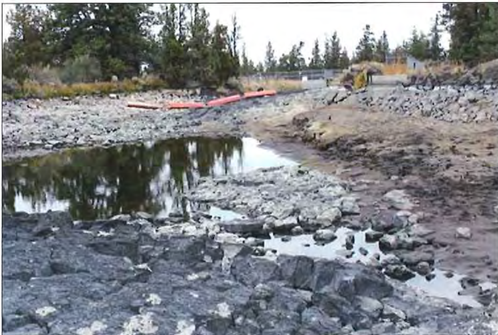
Photo 18 of 19: Segment 5. Approaching northern boundary of historic district. Lava flows, irregular canal bed, irrigation water delivery system slide gate on right. Pink buoys warn of danger ahead, looking north.
