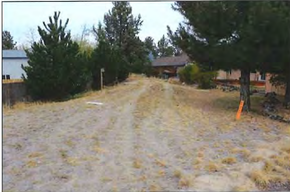
Buried 4' diameter Swalley pipe runs between houses in a residential subdivision in northern Bend, looking north from Cooley Road.
