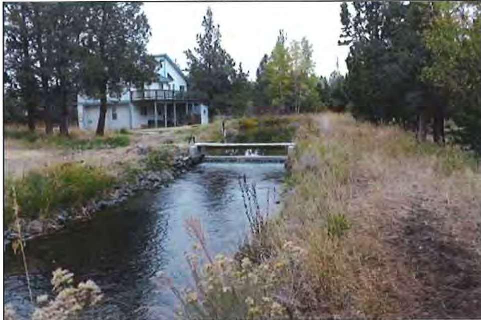
Swalley Canal looking south from Tumalo Road in agricultural area.
