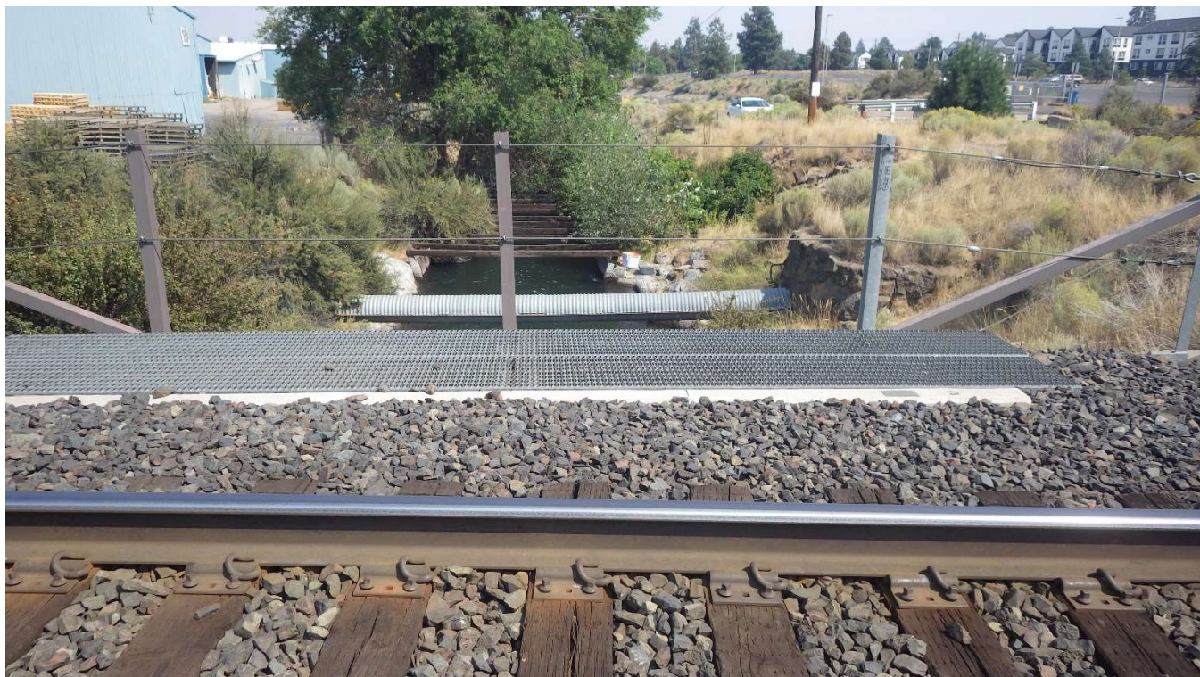
View: OTR/PBC Crossing, Looking East, from OTR Track (G. Kramer, August 2024)
