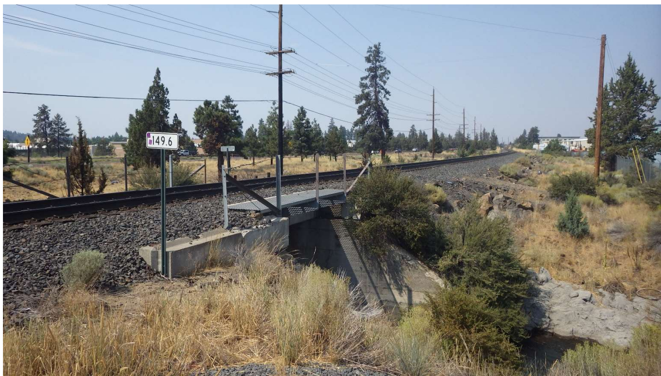
View: OTR/PBC Crossing, Looking Northwest from COID/PBC Maintenance Road (G. Kramer, August 2024)
