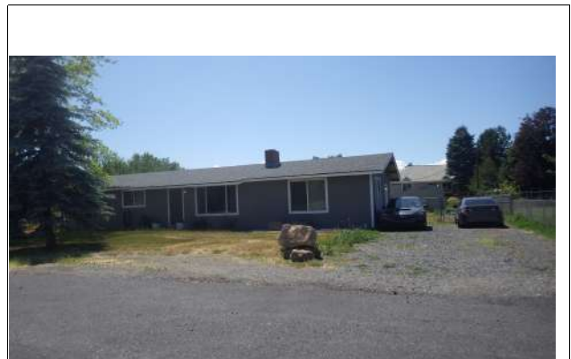
Looking SE from 26th Ave
