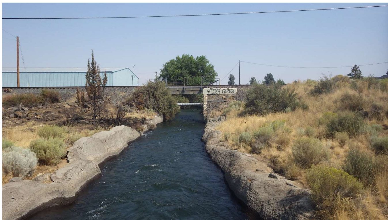
View: OTR/PBC Crossing, Looking East from US 97 Onramp (G. Kramer, August 2024)
