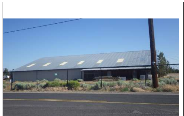
Looking NW from Quarry Ave
