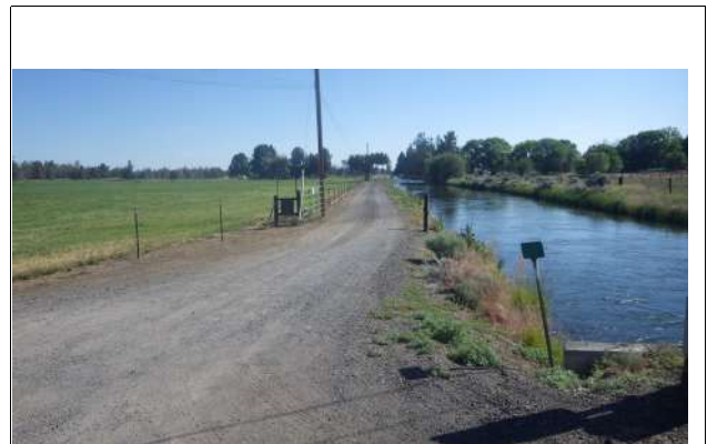
Looking N, from Quarry Ave.
