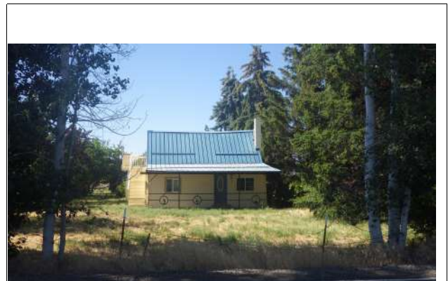
Looking South, from Quarry Ave
