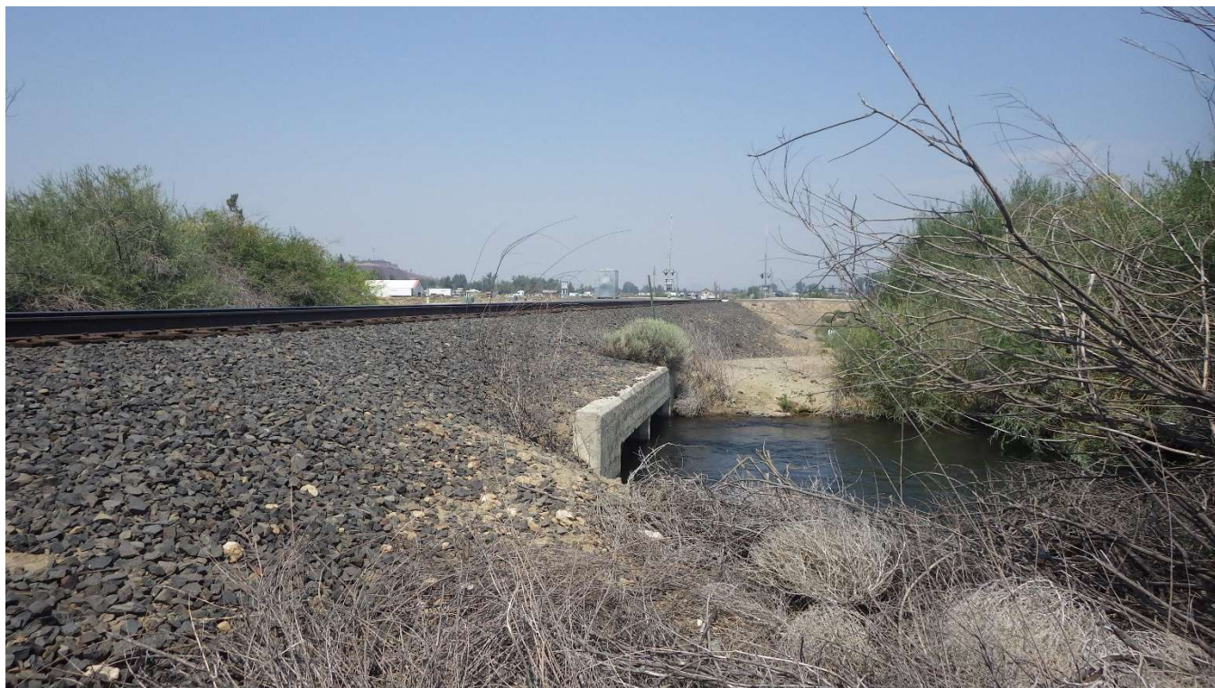
View: OTR/PBC Crossing, Looking NW (G. Kramer, August 2024)
