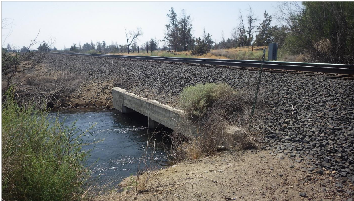
Photograph 2. OTR crossing the PBC at NE King Way.
