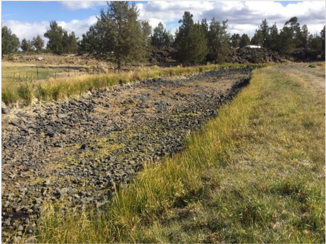
Photograph 4. PBC Alignment in Unincorporated Deschutes County
